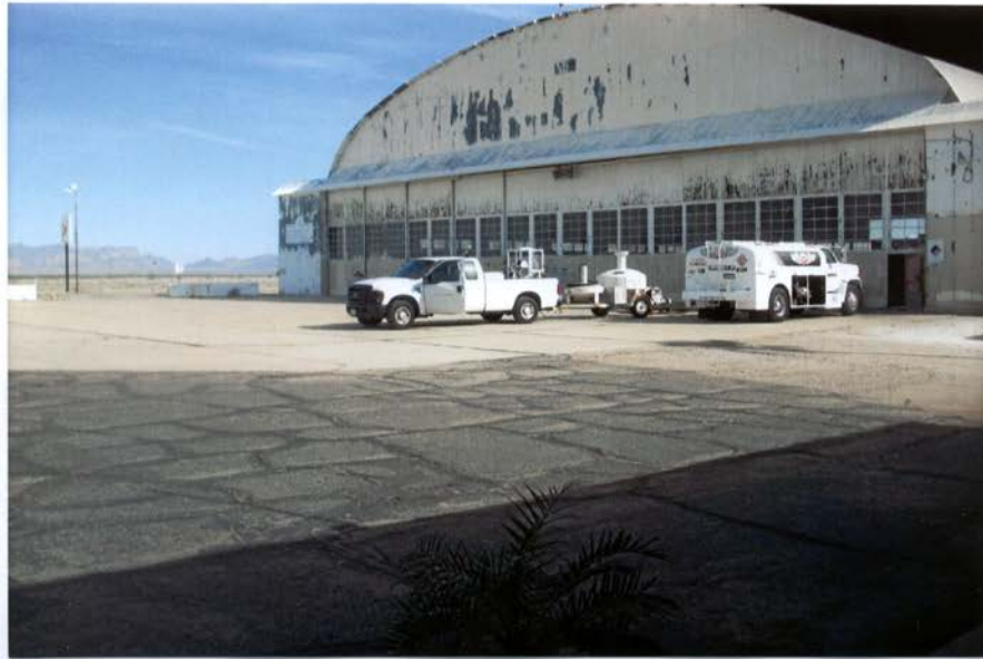
BLYTHE AIRPORT – 1942 HANGAR, FRONT VIEW ATTACHMENT "C"
